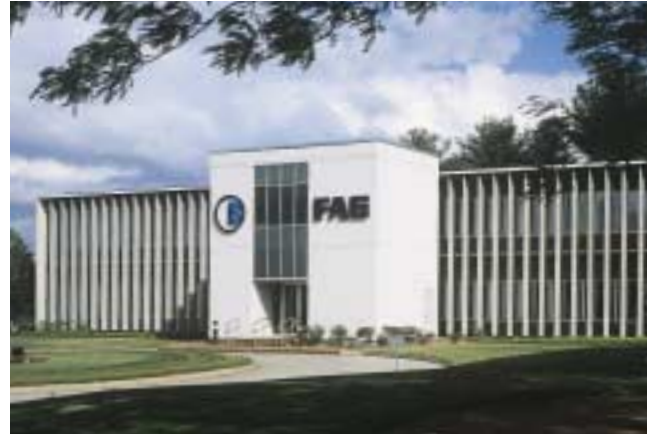
Barden's Super Precision Bearing plant in Danbury, Connecticut.
